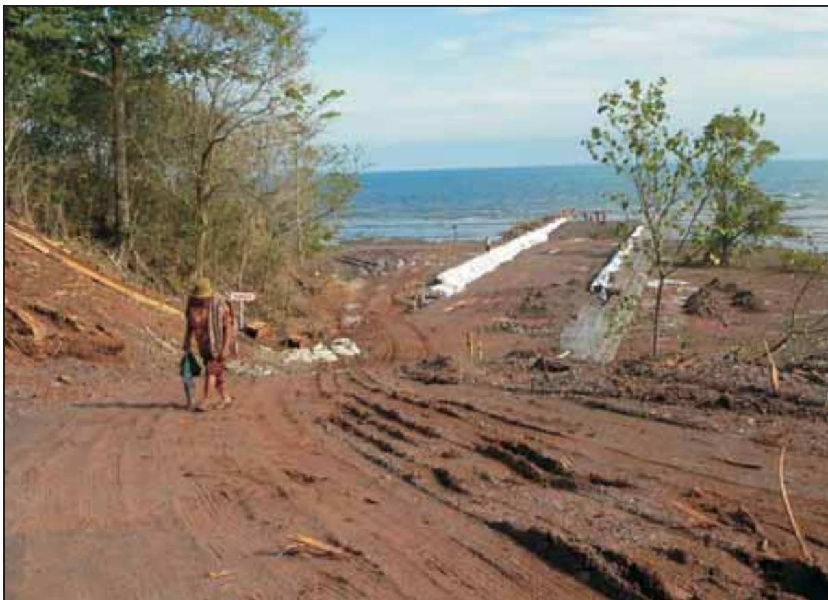
Construction of the port for the Alle-Alle wood chip mill
