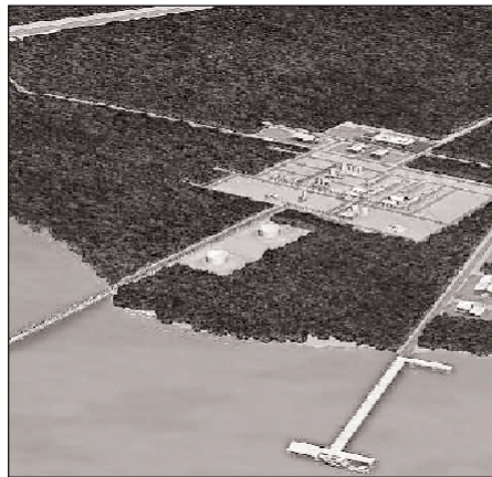
Impression of Tangguh gas installations in Bintuni Bay, in AMDAL
