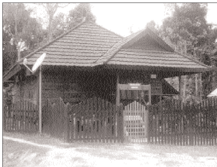
A model house in the new village built for families moved from Tanah Merah village - now the site of Tangguh's LNG plant in Bintuni Bay, West Papua.
