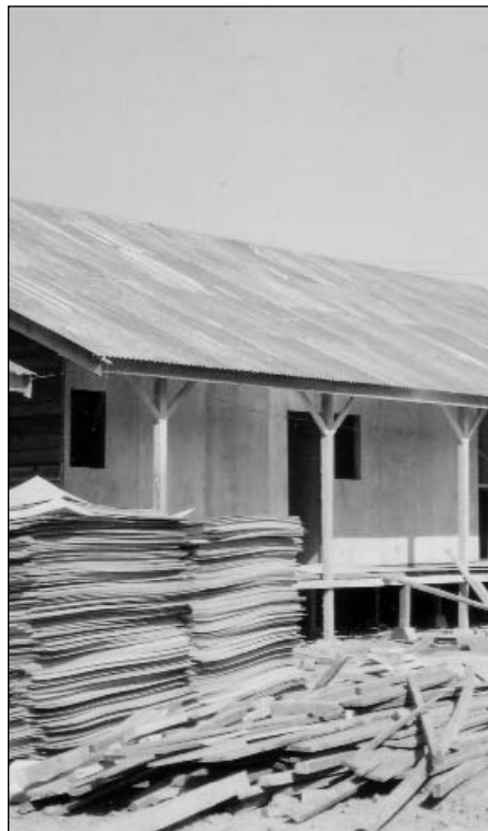
Relocation barrack under construction, early 2005 (DTE)
