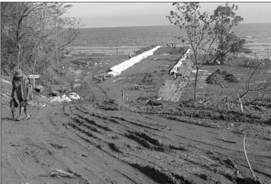
Jetty construction on Pulau Laut, for the UFS chip mill.
